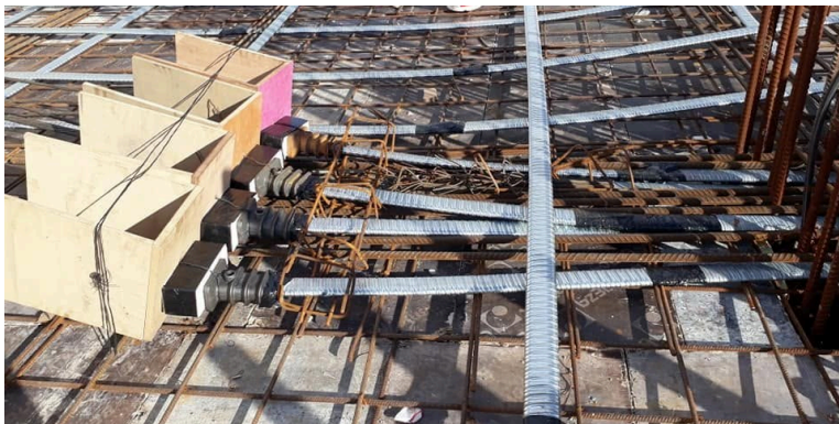
02 Live-end anchorages with bursting spirals.
