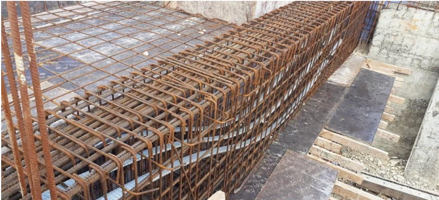
01 PT beam cage with the draped flat ducts, before the pour.
