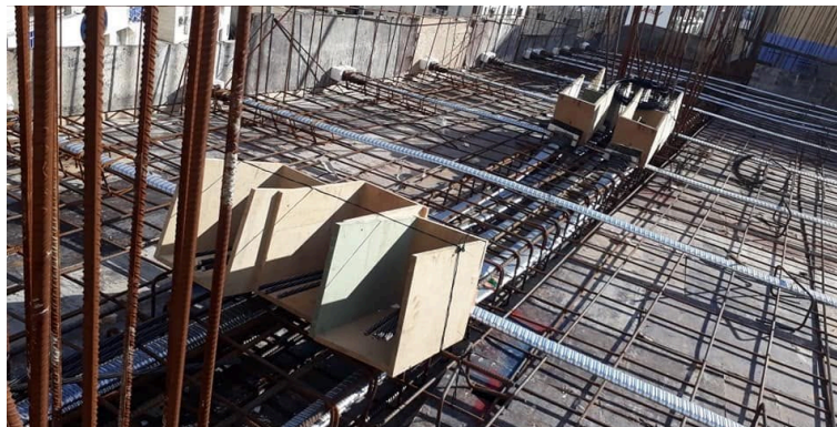
03 Pocket formers at a PT beam end.
